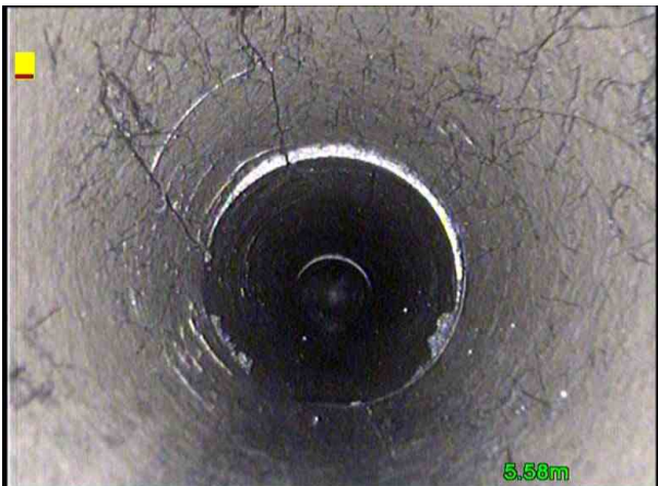
MH1X_2a3f063b-ce7e-4211-8c1e-818aead97839_20190719_090618_887.jpg, 00:00:49, 5.58 m Roots, fine, start
