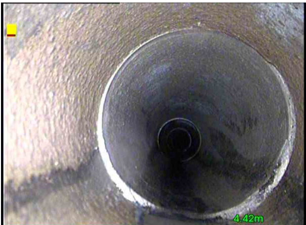
MH2X_2c8affc0-4bb9-47ff-85b6-6fd752258e0d_20190719_091138_243.jpg, 00:00:29, 4.35 m Joint displaced, medium
